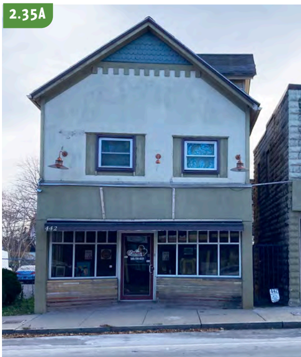
442 North Street (present-day)
