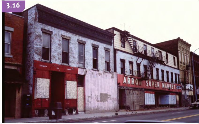
310-314 North Street in 1988 (3 story building with fire escape) (demolished)
