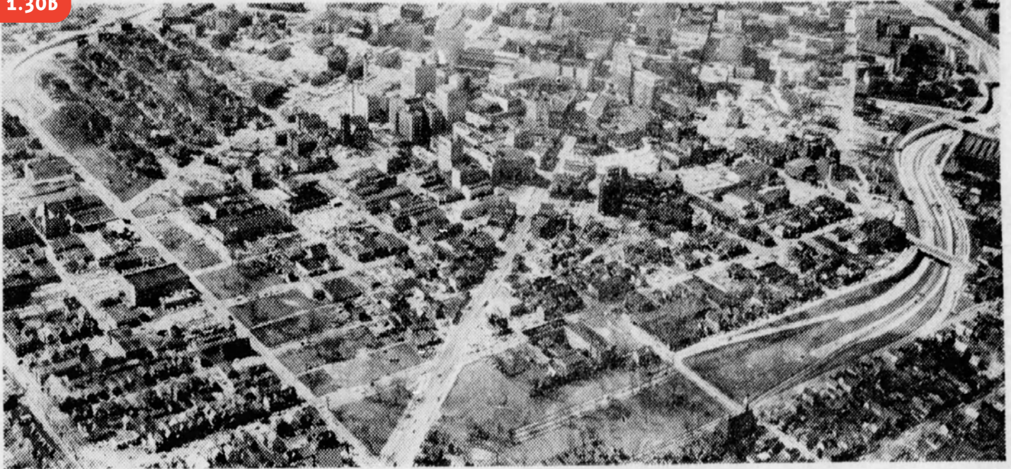
LOOPING THE LOOP—Air view looking over city shows final loop arc. Work starts in two weeks.
