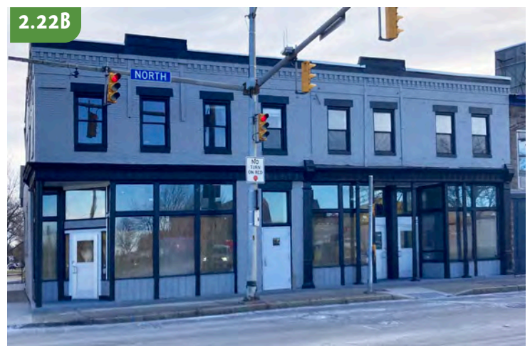
280-286 North Street (present day)
