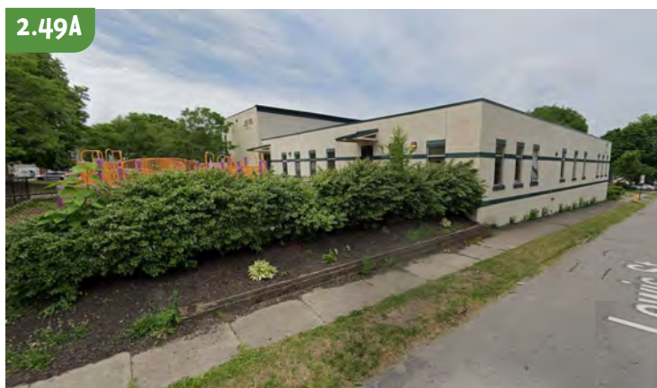
53-57 Lewis Street (present-day)
